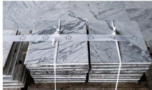
Marble slabs stacked on pallet during deconstruction works. North Station, Brussels. This marble was identified as a specific Carrara variety called Arabescato. Photo: Rotor.
