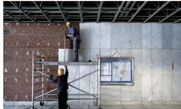
Removal of marble slabs at the North Station in Brussels during a 2018 revamp. Photo: Rotor.
