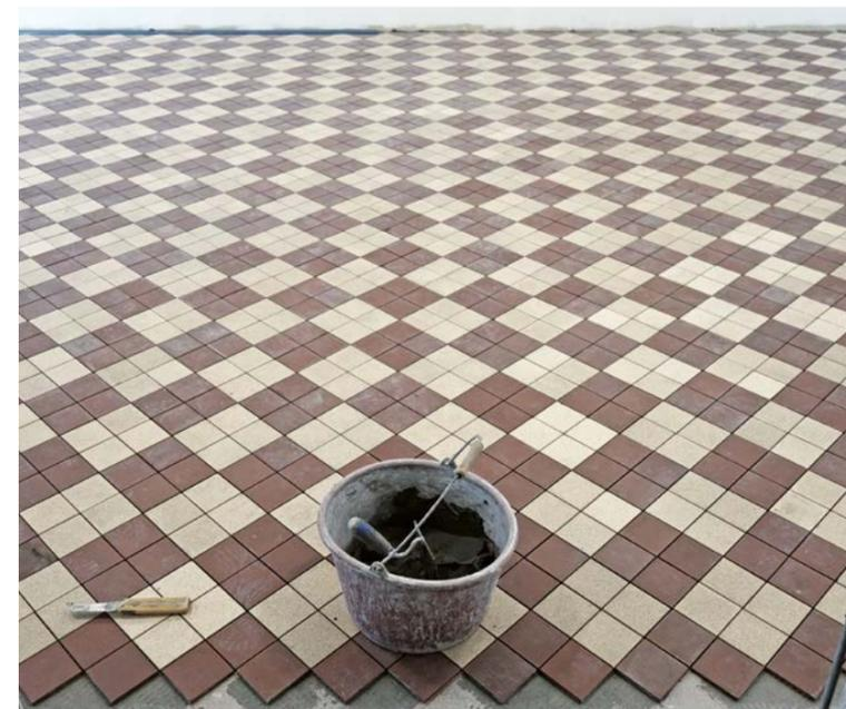
These ceramic tiles, extracted from a 1940 office of the national Telecom company, are being reinstalled on-site after cleaning at Rotor DC. The offices have now become apartments. Tivoli-building, Brussels. Photo: Rotor.
