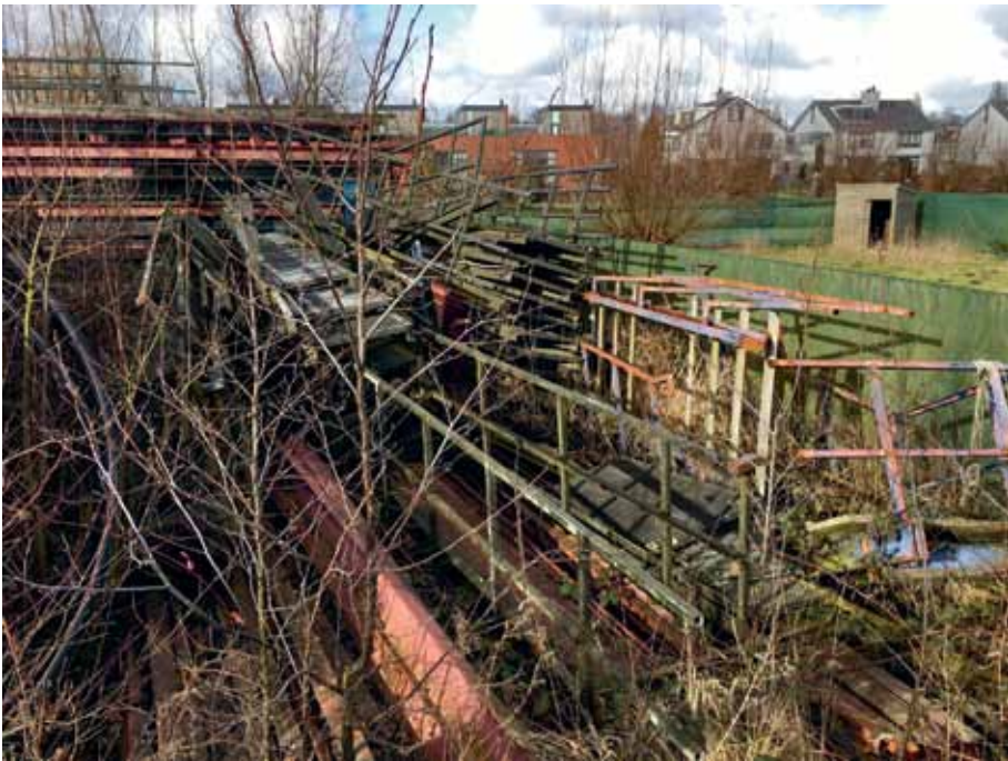
Dismantled steel components of the structure of the former youth hostel in Ockenburgh by Frank van Klingeren, removed and stored in 2010.
